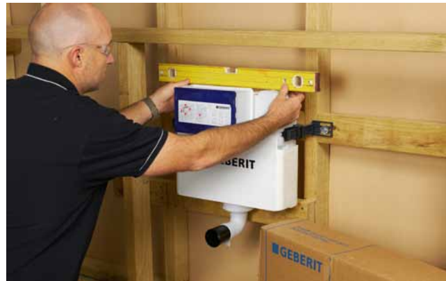
Adam Powell is installing a Geberit Kappa under counter concealed cistern.
